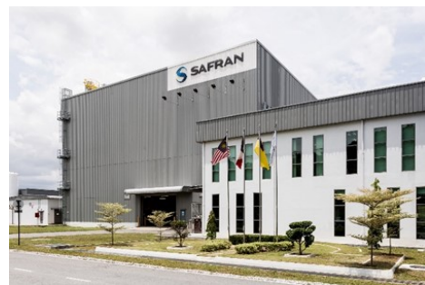
Safran facility in Sendayan
